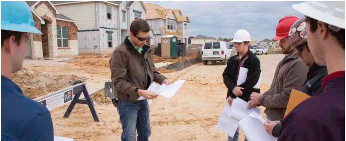
Ryan Day '12, a Land Development Project Manager with PulteGroup, leads a group of construction science students on a tour of a subdivision under con-
