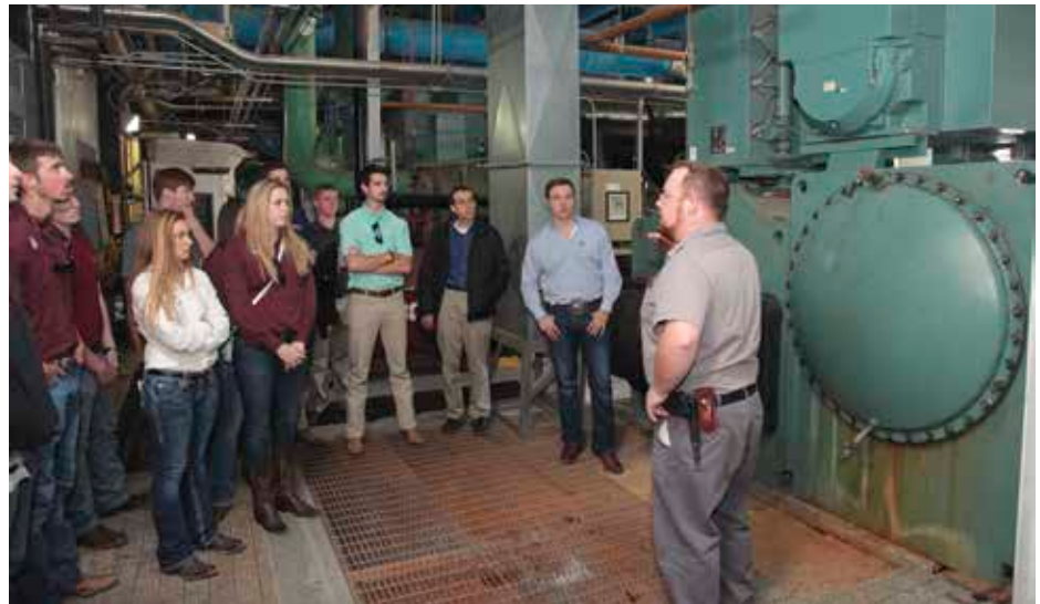
Construction science students visit a physical plant on the Baylor University campus during spring 2015 field day. Students also visited Baylor's football field and other new facilities. During field day each semester, students choose one of several sites that reflect the latest construction, material production and manufacturing practices.
