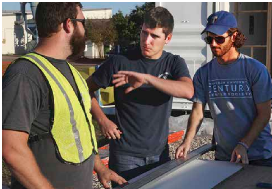
Scott Parshall, left, and Martin Montgomery, center, were among the many construction science students who helped BUILD, a student service organization, convert four shipping containers into mobile medical clinics.
